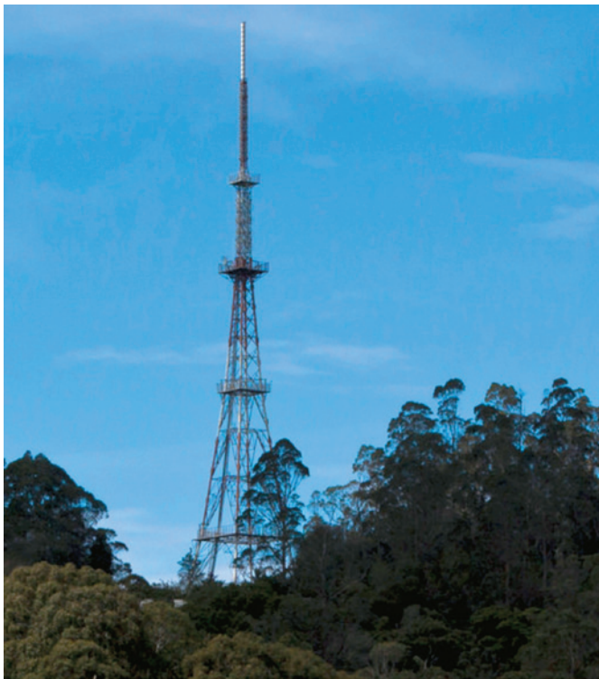
Figure 3: 150m TV Tower Kodaikanal
