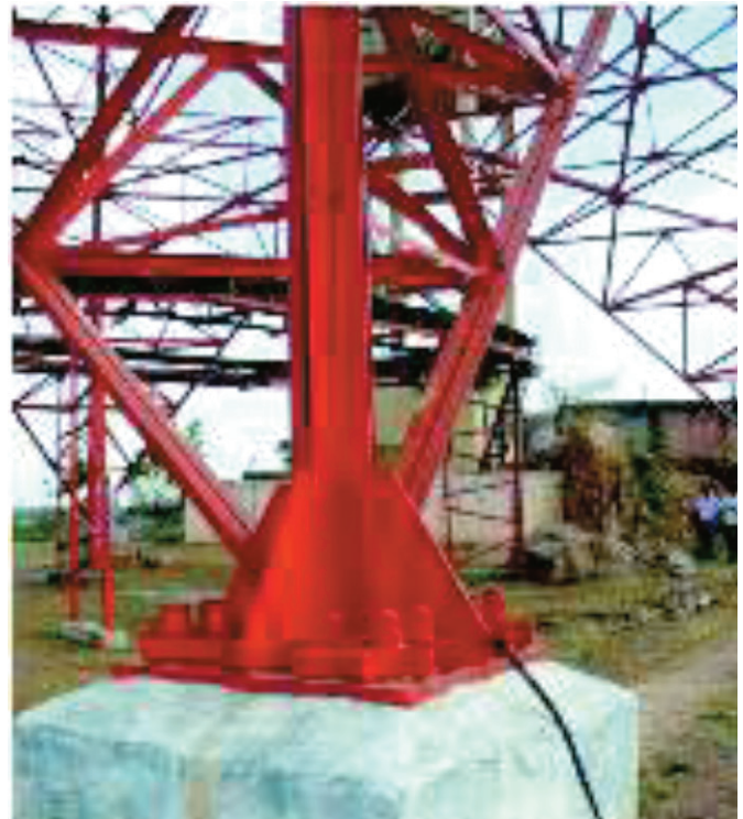
Figure 1: Typical self-supporting tower base
