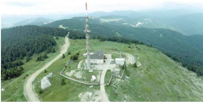
An example of TRT Transmitter Station
