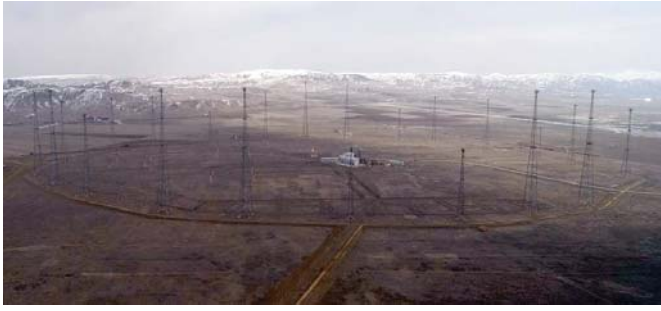
Short Wave Transmitter Station
